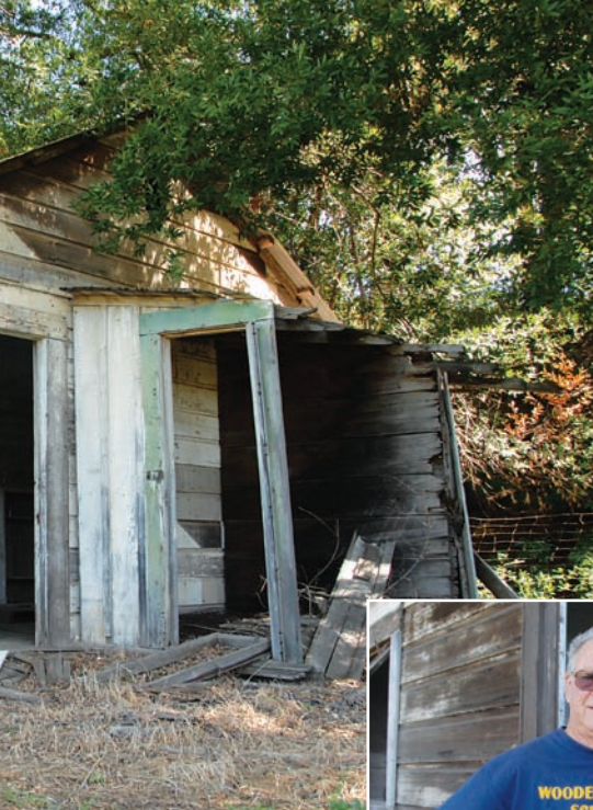
LEFT: The former Wooden Valley School, a one-room schoolhouse in Napa, no longer in use.
